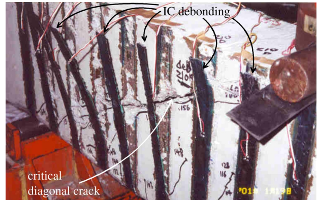
Fig. 1. IC debonding of transverse FRP plates [9].
