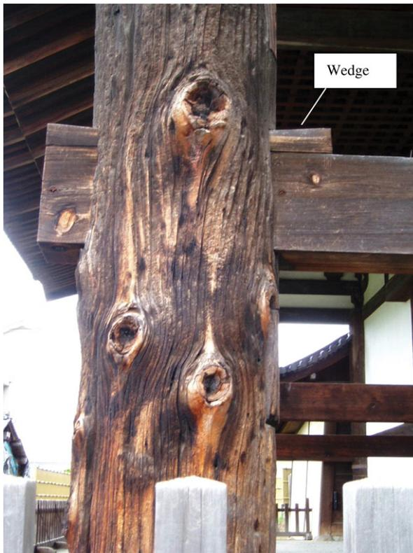
Fig. 1. A typical ‘Nuki’ joint in a traditional Japanese temple.
