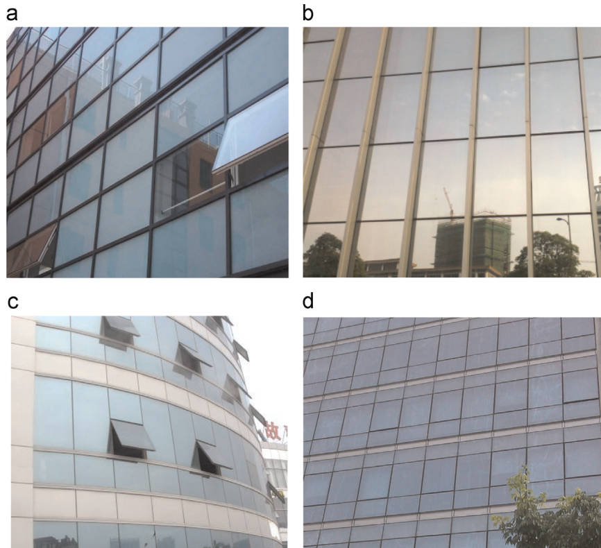
Fig. 1. The frame supported glass curtain walls, photographed in four cities in China. (a) Exposed frame, Suzhou; (b) Horizontal-hidden frame, Hefei; (c) Vertical-hidden frame, Huainan and (d) Hidden frame, Shenzhen.
