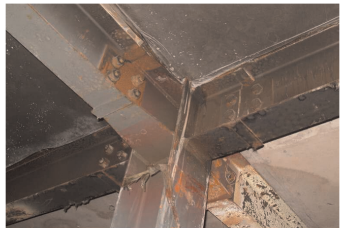
Fig. 2. Picture of the beam-to-column connection.
