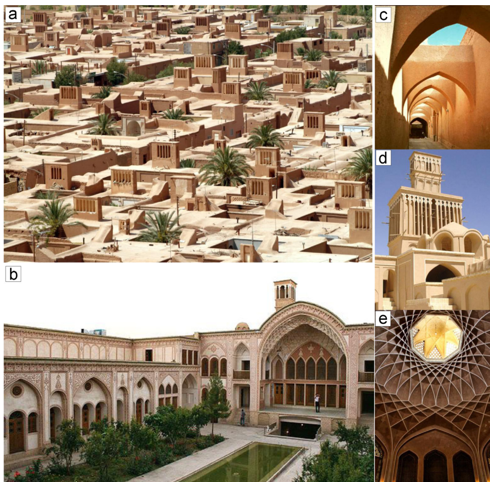
Figure 1 Environmental sustainability of traditional courtyard houses in the hot and dry climate of Iran: (a) compact urban layout of the structure of the Chupanan Desert town, Isfahan; (b) traditional courtyards as microclimate modifiers, Kashan; (c) narrow enclosed alleys provide shade during summers, Yazd; (d) traditional wind catchers as natural cooling systems, Yazd; and (e) roof dome windows provide natural light, Kashan (Soflaei, 2004).
