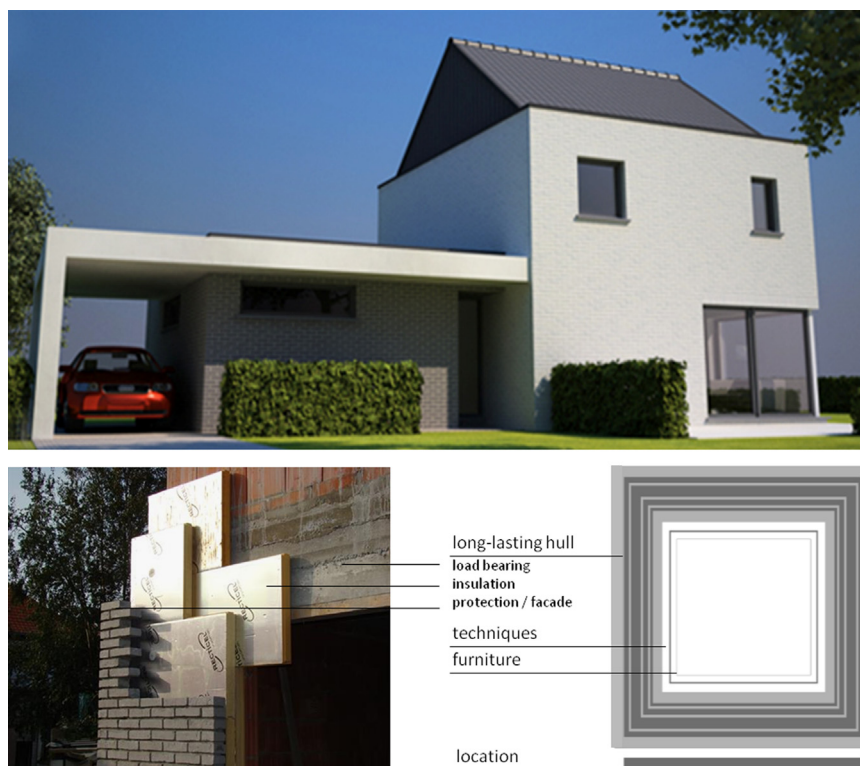
Fig. 1 Reference house with detail of the outer wall, showing the functional layers of the house in a theoretical composition, displaying their durability (line weight) and interrelationship (overlap). (design/photo: arch. Cauchie).
