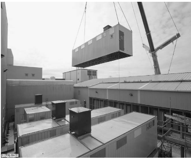
Fig. 2. Installation of the last power Unit of ERFA.
