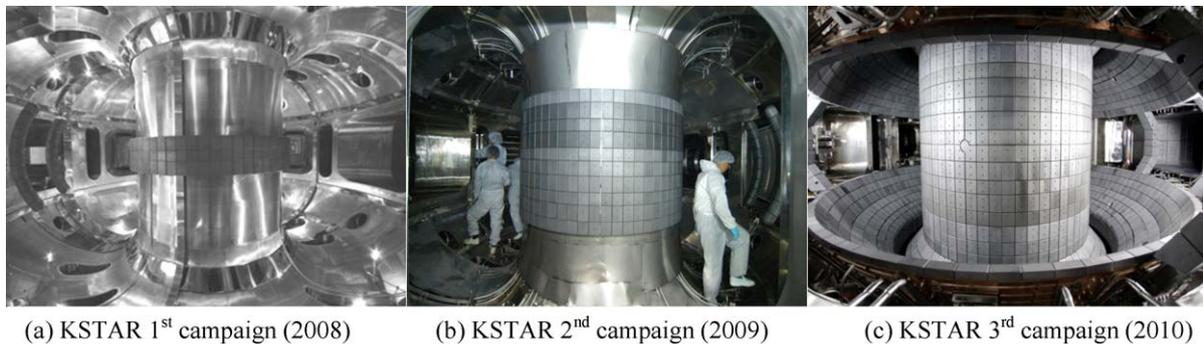
Fig. 1. Step-by-step installation of Plasma Facing Components from 2008 to 2010.
