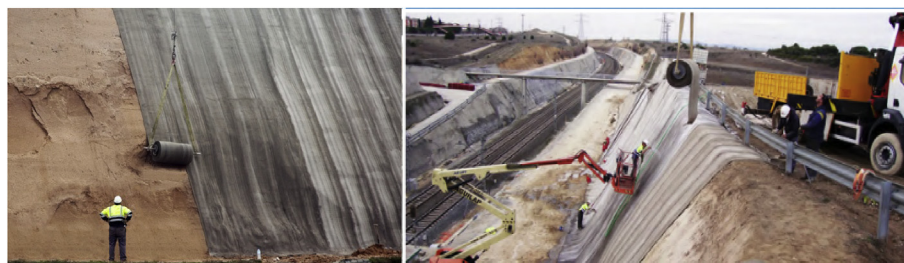
Fig. 2. Concrete Canvas is rolled off a crane to stabilize a slope (Photo courtesy of Concrete Canvas Ltd.).
