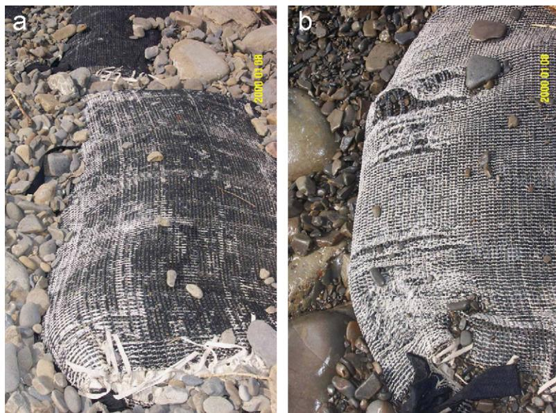
Fig. 2. Various degrees of damage to the geogrid containers observed 1 month after completion: (a) example of moderate damage and (b) example of serious damage.
