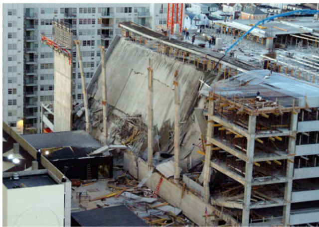
Fig. 1 Progressive collapse of Tropicana Casino parking garage due to punching of flat slab [3].
