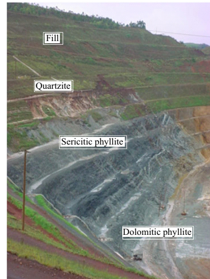
Fig. 2. Partial view of east portion of the slope, in February, 2005 [4].
