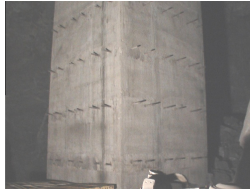
Fig. 4. View of concrete pillar in Fetra6 underground mine.
