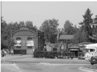
Fig. 2. View of the buildings of the hoisting machine and shaft top.
