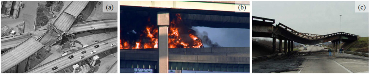
Fig. 1. (a) MacArthur Maze fire in Oakland, CA [1], (b) I-81/Rt 322 interchange fire in Harrisburg, PA [21], and (c) malfunction junction fire in Birmingham, AL (photo courtesy of Alabama Department of Transportation).
