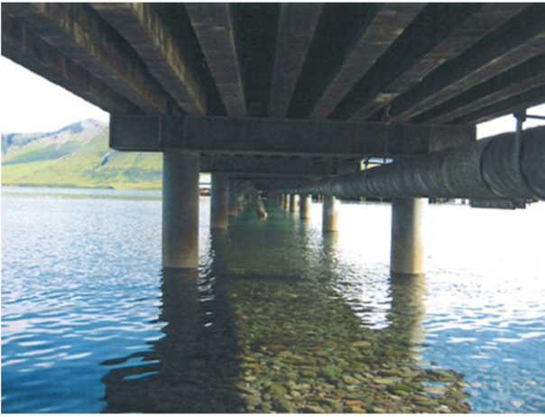
Fig. 1. Driven steel pile bridge pier. Courtesy of AKDOT.
