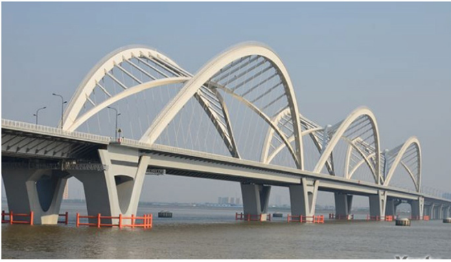
Fig. 1. Main navigational structure of the Jiubao Bridge, Hangzhou, China.
