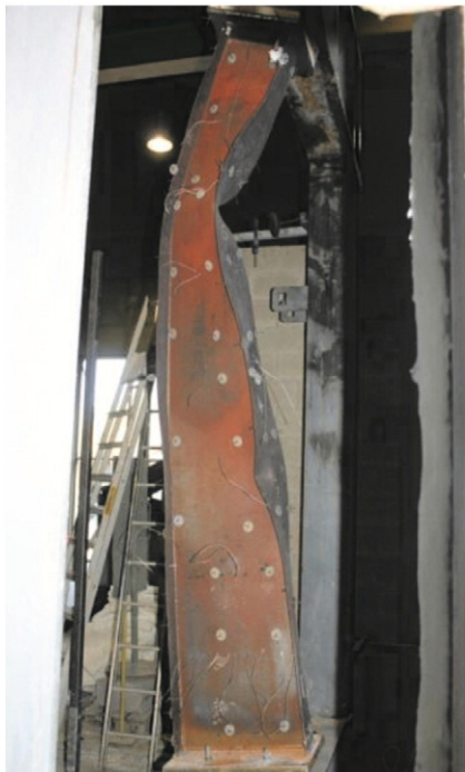
Fig. 2. Example of column showing local buckling from a test performed at elevated temperatures at the University of Liège (taken from [13]).
