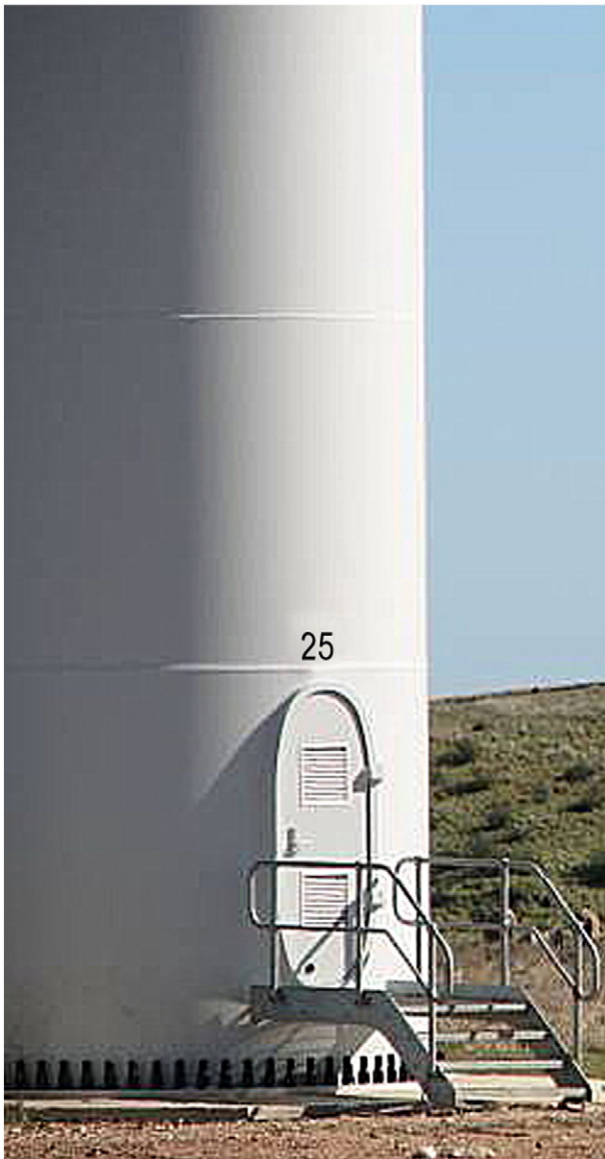
Fig. 1. Entrance door of a wind turbine tower [8].
