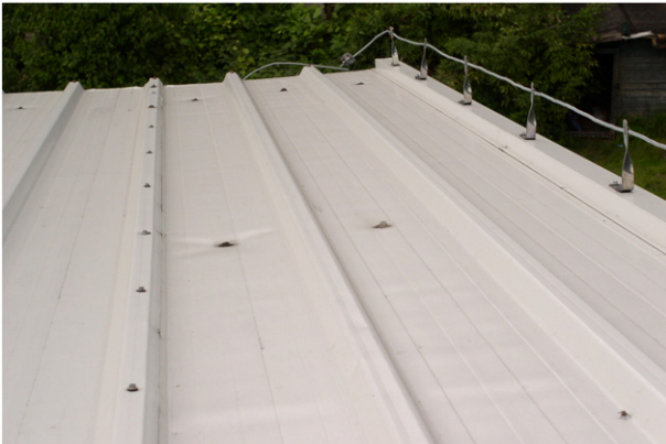
Fig. 2. Roof covering from sandwich panels with deep-profiled upper facing and low-profiled bottom facing.
