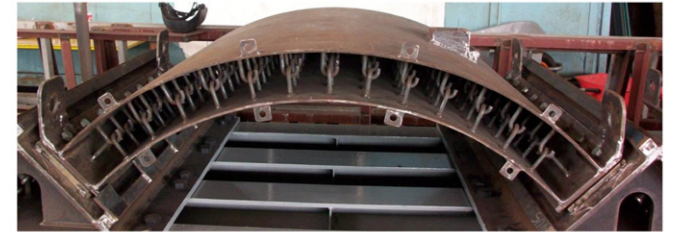
c) SCS sandwich shell with the J-hook shear connector (before casting)
