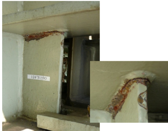
(c) Fatigue crack
