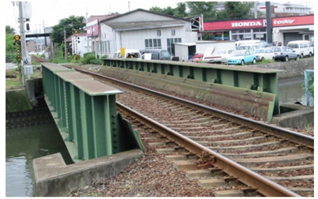
Fig. 2. An old steel railway bridge.
