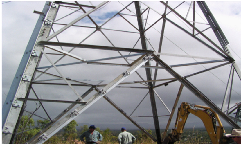
Fig. 1. An example of a reinforced tower leg installation underway in Australia (photo from Graham Brown, O'Donnell Griffin Pty Ltd).
