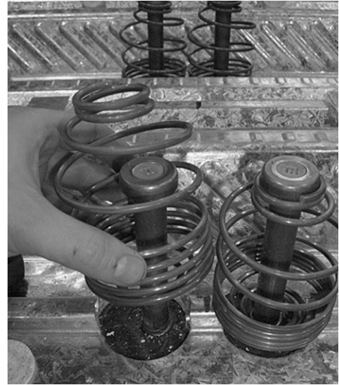
Fig. 1. Stud performance-enhancing device being fitted around a stud and finally clipped under the stud head.
