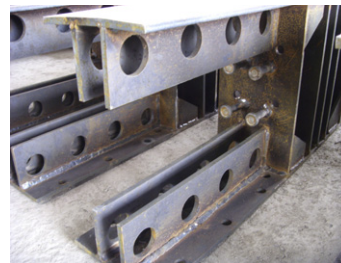
Fig. 2. New mixed girder and connection detail.
