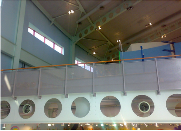
Fig. 1. Practicality of cellular beams in constructing various elements of main structural systems.
