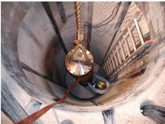
Fig. 2. Installation of the canister retrieval test.
