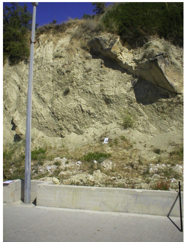
Fig. 4. “Cantilever” of harder sandstone layer on the slope (differential weathering along the slope).
