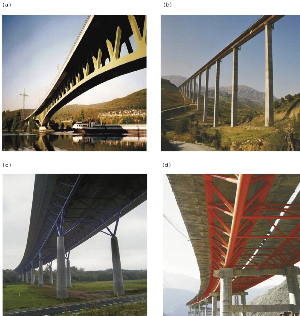
Fig. 1 – Typical composite bridges. (a) Nantenbach Railroad Bridge (Germany). (b) Arroyo Las Piedras Viaduct (Spain). (c) St. Kilian Viaduct (Germany). (d) Ganhaizi Bridge (China).
