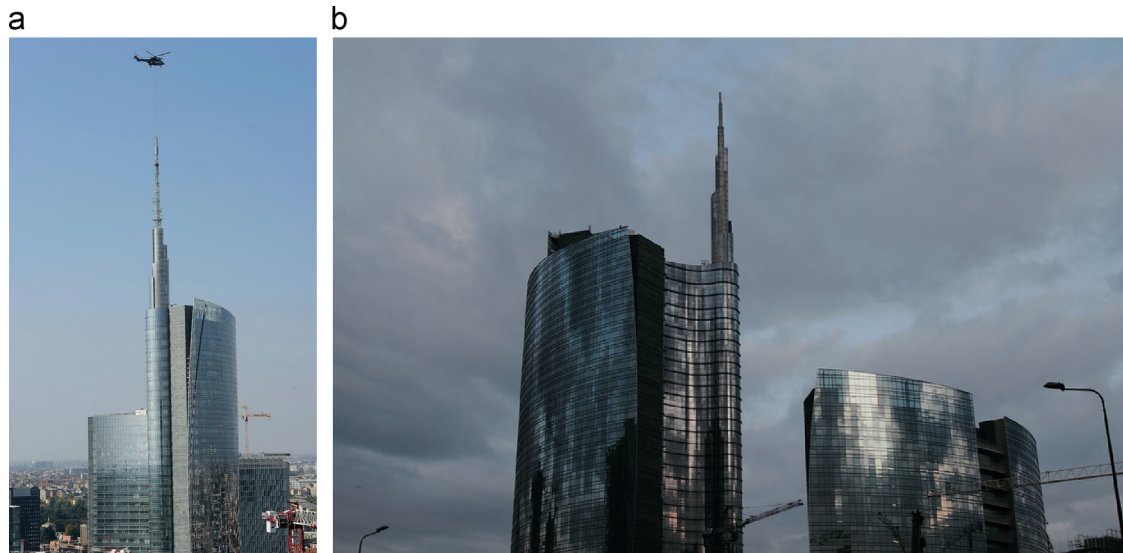
Fig. 1. The 139 m tall spire object of this study. (a) The bold final stage of its erection. (b) The final structure.
