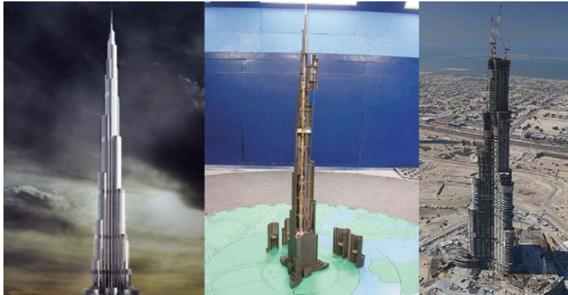
Fig. 1. Burj Dubai—future view, aeroelastic model and recent construction photo.
