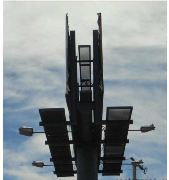
Fig. 3. Back to back thin plate sign.
