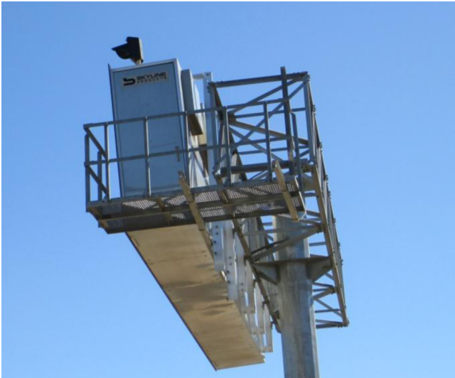
Fig. 1. Sign with significant thickness.
