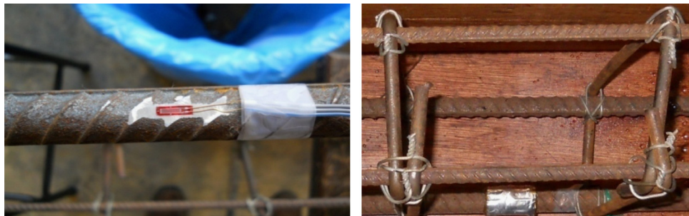
Fig. 2. Installation of strain gauge (Left) and strain gauge protection (Right).
