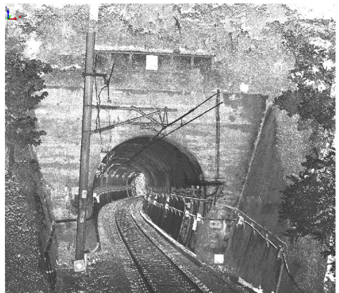
Fig. 1. Scanning results illustrated by using backscattered intensity of the Jipyung tunnel.
