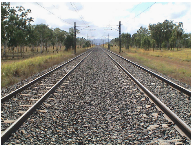
Fig. 1. Typical ballasted track on a coal line in Central Queensland (after [7]).
