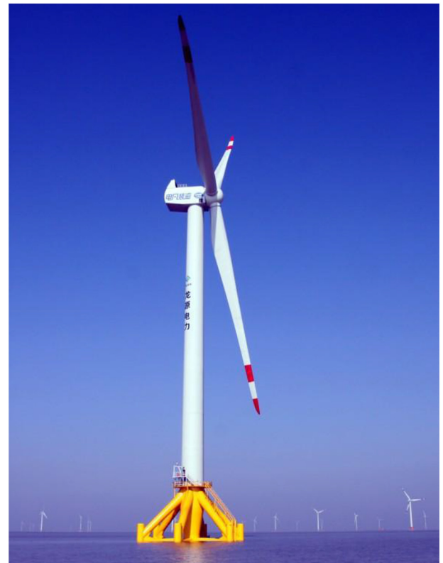
Fig. 2. 5 MW wind turbine.
