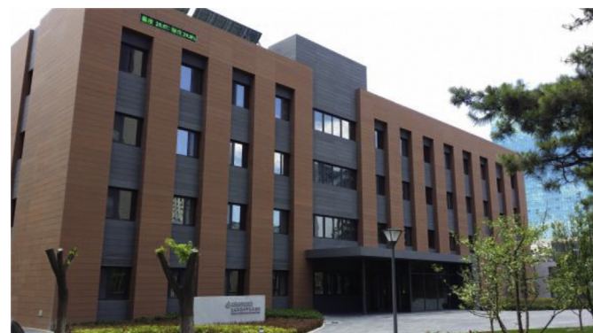
Fig. 1. Outlook of the nearly zero energy building.
