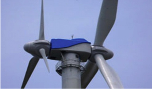
Fig. 1. Dual-rotor wind turbine.
