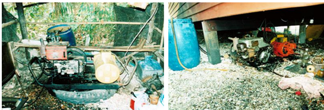
Fig. 1. Electricity supplied by diesel generators before the installation of the PV hybrid system.
