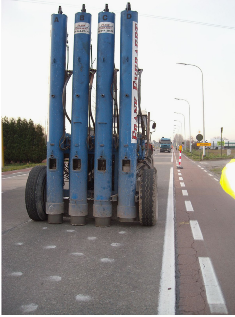
Fig. 1. Multi-head pavement breaker used for fracturing of the concrete roads.
