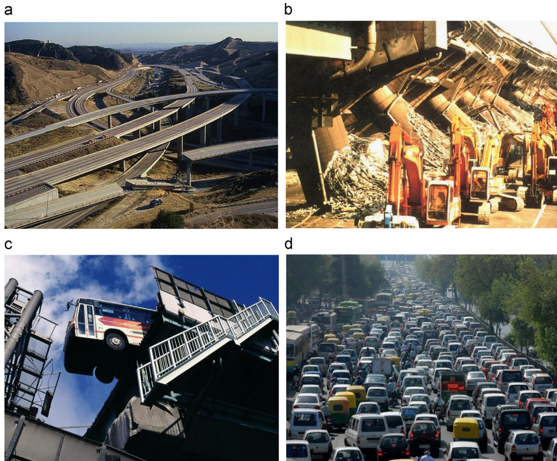
Fig. 1. Structural damage of motorway bridges during: (a) the 1994 Northridge earthquake, and (b) the 1995 Kobe earthquake; (c) bus traveling on Hanshin Expressway Route No. 3 marginally stopping before a collapsed bridge span; and (d) deterioration of serviceability due to closure of road segments.
