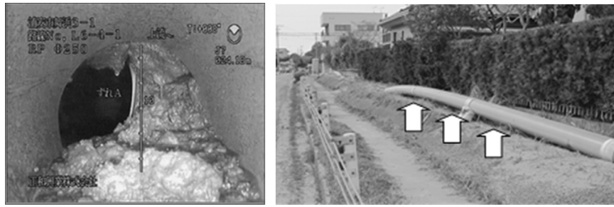
Fig. 1. Clogging and floating of embedded pipes.
