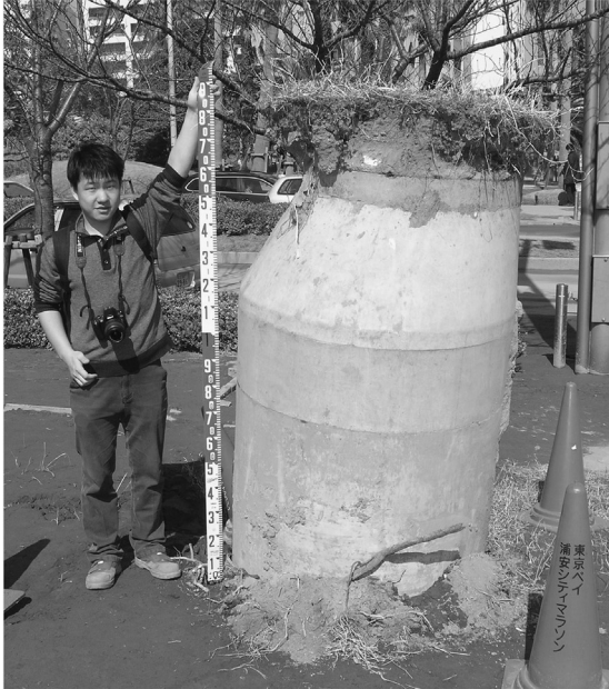
Fig. 1. Examples of liquefaction-induced damage in sewage facilities: (left) floating of manhole and (right) clogging of sewage pipes.
