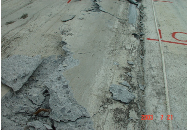
Fig. 1. Extrusion damage to concrete face slabs in Tianshengqiao-1 CFRD project.
