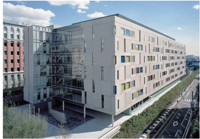
Photo 1. View of 7-story office building in Shinsuna.
