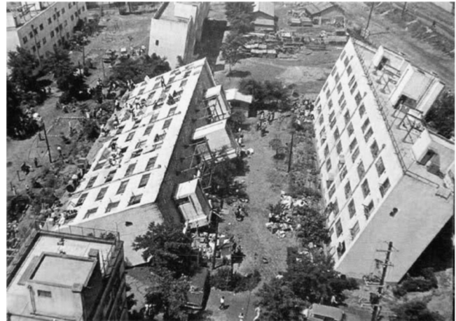
Fig. 1. Tilted apartment buildings in Niigata (Niigata Nippo Newspaper, 1964).
