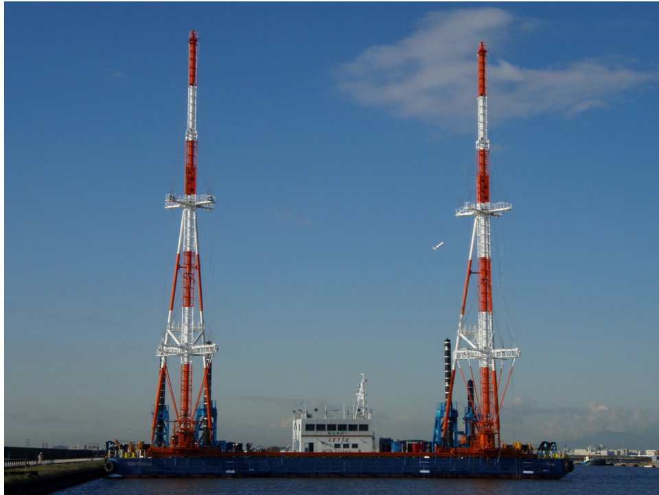
Photo 1. PVD installing machine on work vessel.
