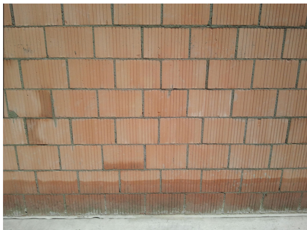
Fig. 1. Typical clay block load-bearing masonry wall.
