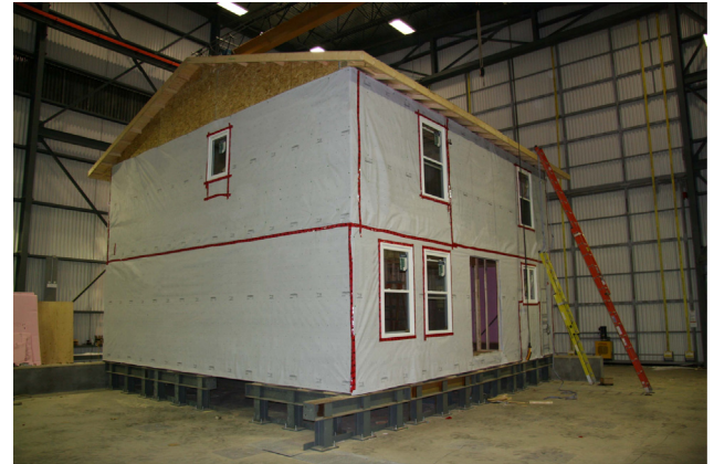
(a) Full scale test house during construction (processed to avoid commercial contains)
