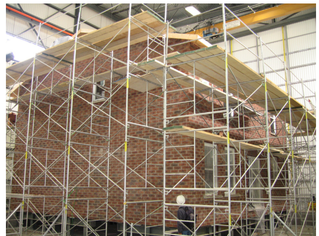
(b) Full scale house after installing brick veneer walls.
